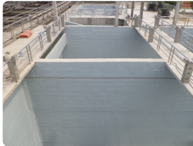
- Clean, wrap the expansion bar - Apply Revinex bonding agent (mix with water in a ratio of 1:4)
