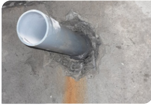
Chamfer around the neck of the pipe
