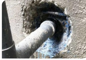
- Clean, wrap the expansion bar - Apply Revinex bonding agent (mix with water in a ratio of 1:4)
