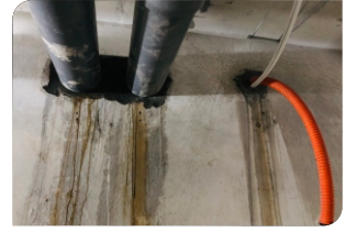
Patch and finish the surface with Neorep repair mortar
