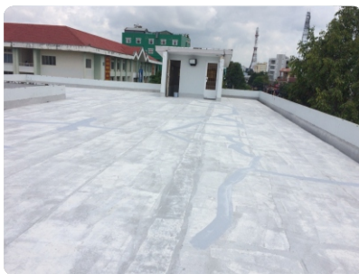
Step 1: Clean concrete surface before construction
