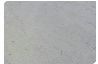
Concrete surface achieved
