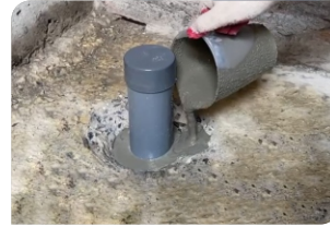
Grouting Construction Lemax Grout LM-G650
