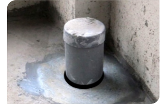
BS 8620S Sealant Injection around Pipe Neck
