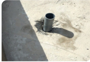
Chisel around the pipe neck, insert foam or formwork below the pipe neck
