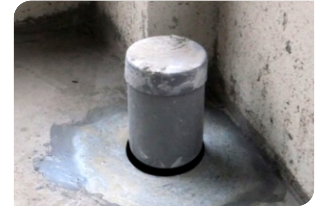
BS 8620S Sealant Injection around Pipe Neck
