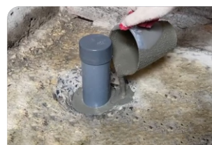
Grouting Construction Lemax Grout LM-G650
