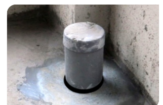
BS 8620S Sealant Injection around Pipe Neck
