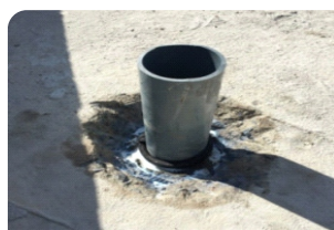
Clean the neck of the pipe, wrap the expansion bar
