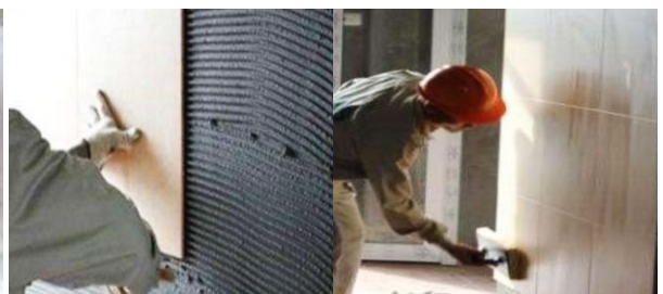
Application of tiles and filling joints
