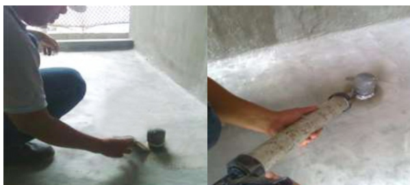
Applying of floor penetration tube stock
