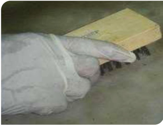
Cleaning surface for preparation
