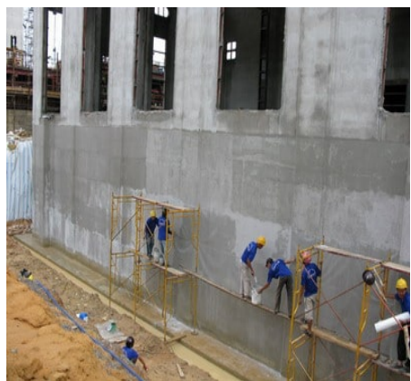
Finish Surface for waterproofing
