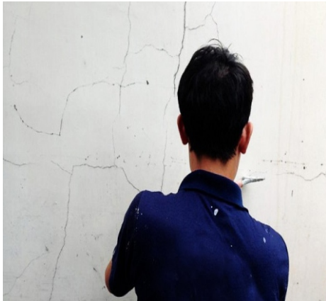
Cut, chisel longitudinally the crack
